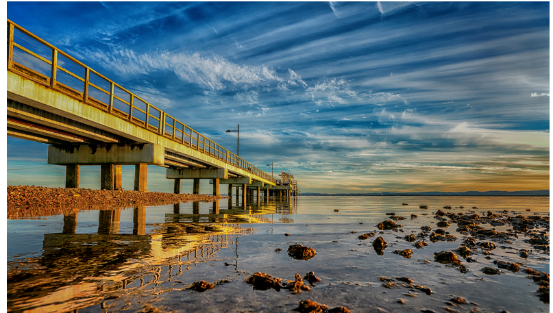
Woody Pt Jetty Merit Peter Simmonds
